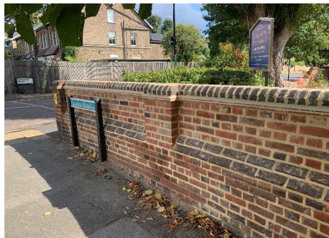
Matching bricks and careful re-pointing restore the Church of Good Shepherd wall in Handen Road
