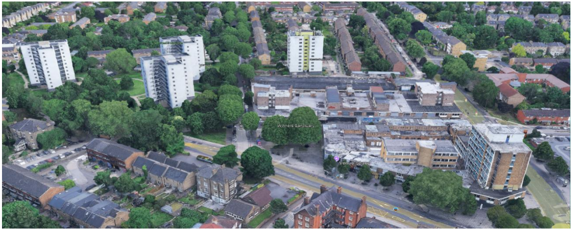
Birdseye view over Leegate site (to the right) showing both the Leybridge Estate (left) and the Carston Close high-rise building (top centre).
